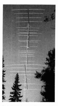
fig. 1. The "Christmas tree" antenna at the contest site of Marty, OH2BH. Six-over-six elements on 20 meters, backed up by single six-element beams on 21 and 28 MHz are mounted on the 170-foot high tower. The 20meter beams can be switched in combinations from the operating position.
